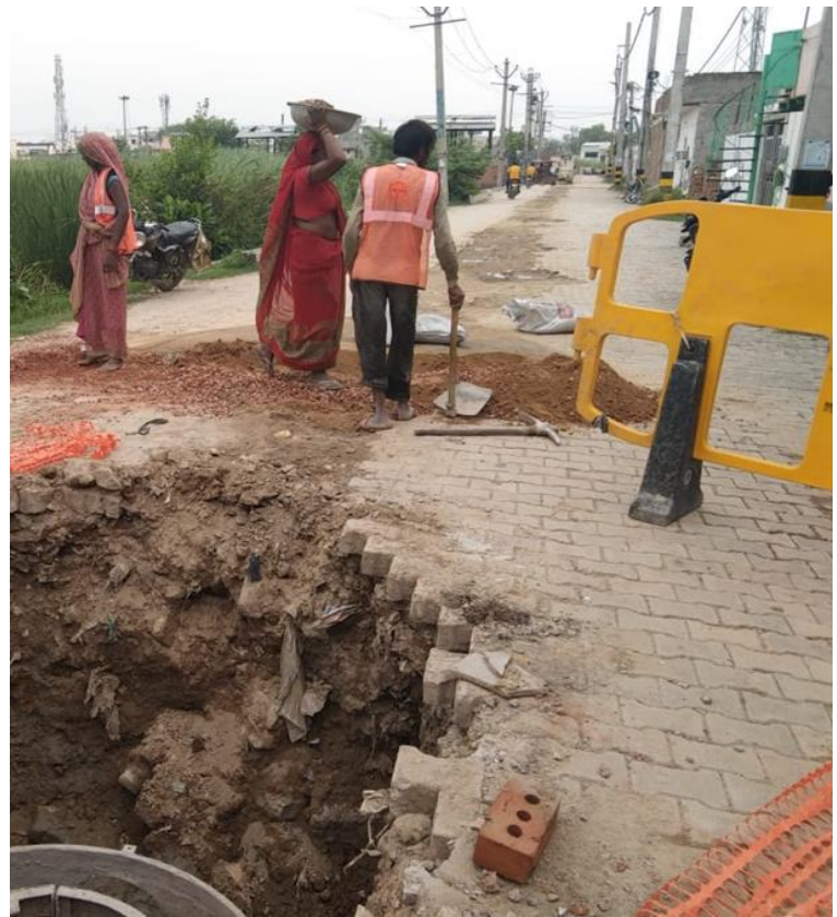
Laying of sewer line - In process
