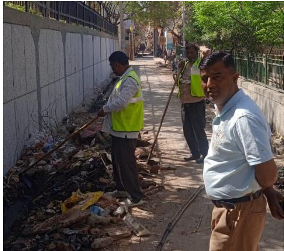
On-going drain cleaning work in G-block, Bakkarwala
